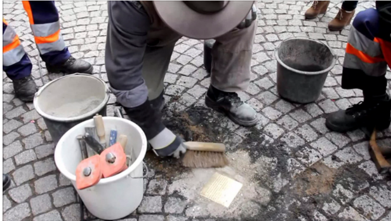
Re-laying the Original Stolperstein. Köln, Germany. 2013.
